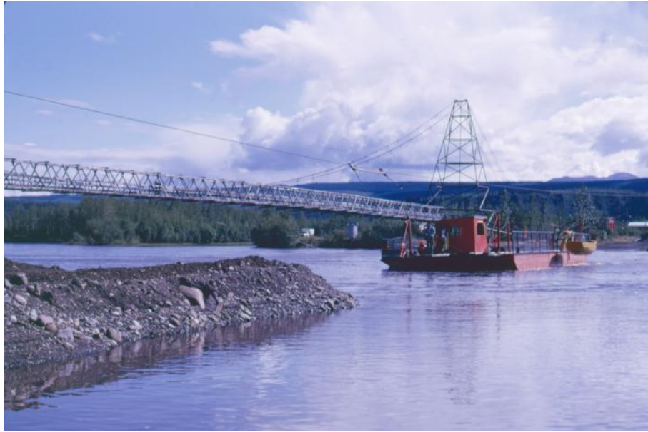
Ross River Suspension Bridge and Ferry, (July) 1970. YA #012364, Gordon and Lorna Walmsley fonds
